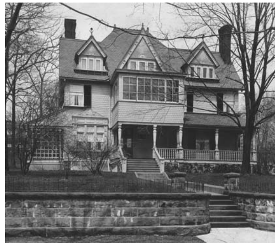
216 Ridgewood Avenue – showing still existing retaining wall
