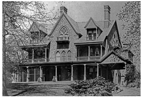
The Darwin family home was a large, eclectic structure mixing rural French and Victorian Gothic forms. The gray rubble stone of the walls was quarried in the Oranges. The rubble walls are reinforced with brick at corners and at openings. The roof was a mix of rectangular and hexagonal slates of uniform color, organized into subtle horizontal bands. The dormer gables were ornamented with wood shingles.
